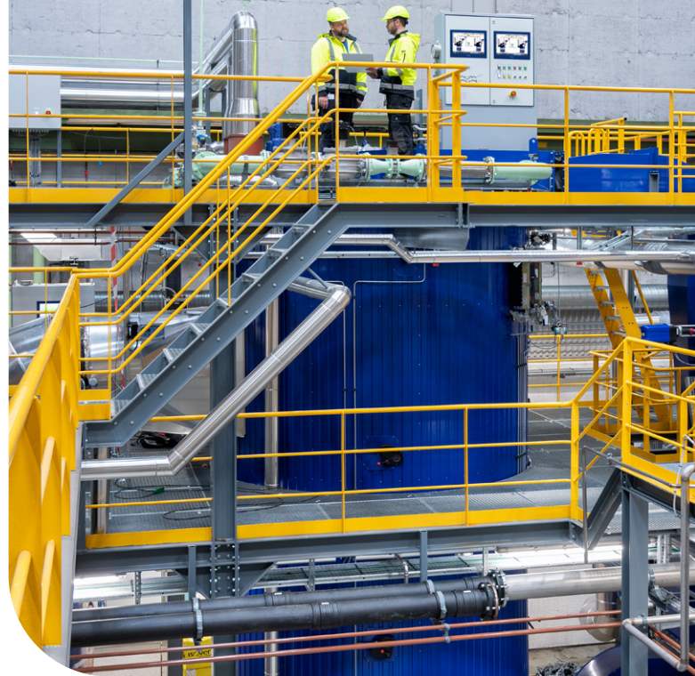
The Alfa Laval Test & Training Centre in Aalborg, Denmark, includes facilities for testing both gas-related solutions and biofuels. It is the world's most advanced test centre for environmental and combustion technology for the marine industry.
